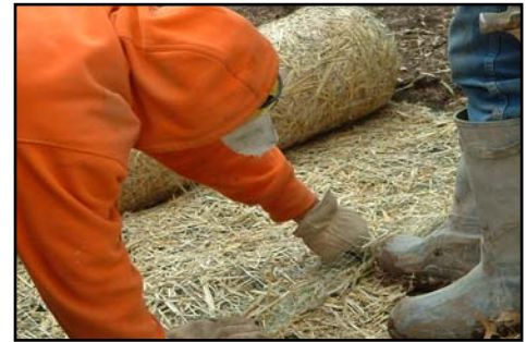
Staking of an erosion control blanket
