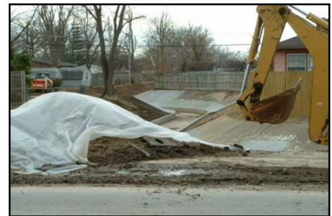
Plastic cover protecting a stockpile from erosion.
