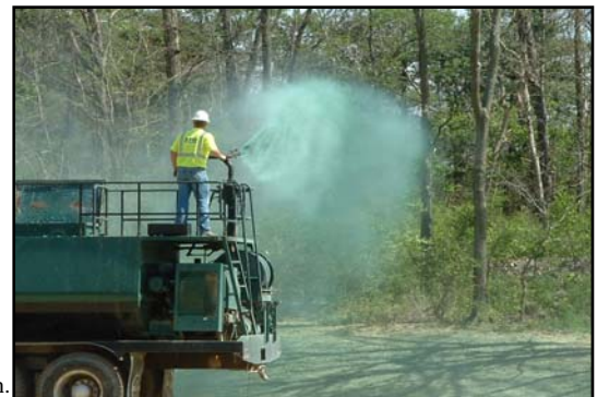
A hydroseeding operation in action.
