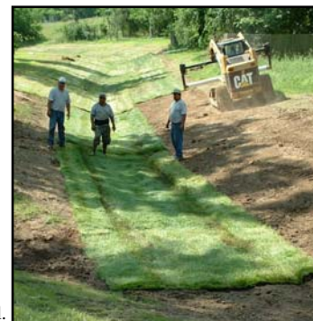
Installation of sod in a grass-lined channel.
