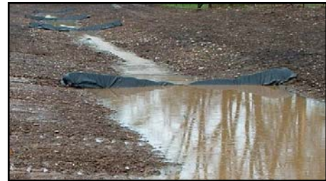
Triangulated silt dikes used as check dams.
