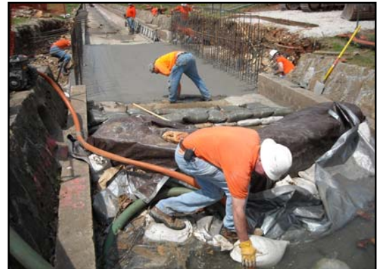
Pumped stream diversion for bridge installation.
