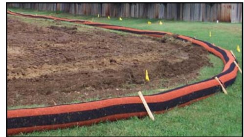
Compost filter sock used as a perimeter control.
