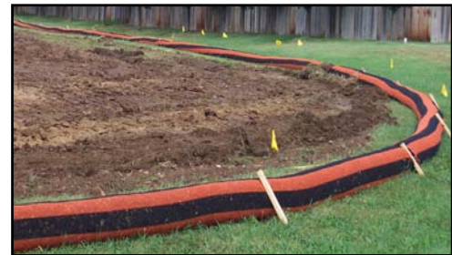
Compost filter sock used as a perimeter control.
