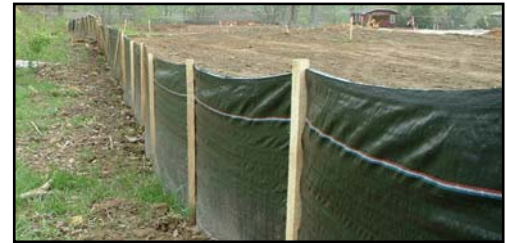
Silt fence used as a perimeter control.
