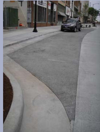
FIGURE 1: PERVIOUS PAVEMENT ON PARK CENTRAL WEST
