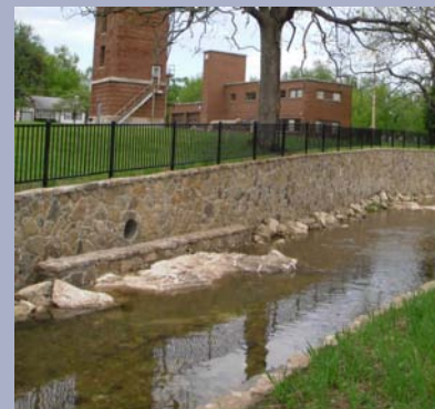
FIGURE 5: RECONSTRUCTED HISTORIC ROCK WALLS
