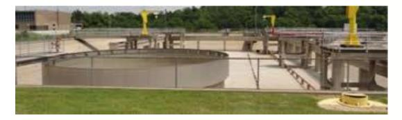
Under these circumstances, 100 million gallons per day receive full treatment while the remainder flows into equalization basins. These basins are capable of holding 41 million gallons. When they become full, the excess diluted wastewater is treated in a peak flow clarifier and discharged to Wilson's Creek.
