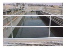
The filter must then be cleaned by forcing clean water through from the bottom of the filter up through the filter media which washes the solids out of the filter. The dirty backwash water is pumped to the head of the plant for retreatment.
