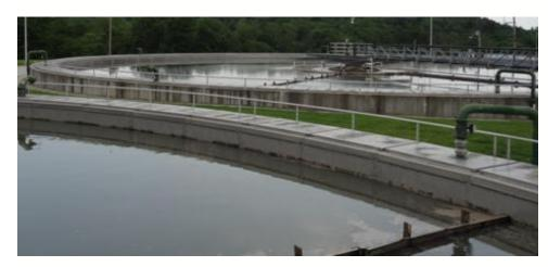
The scrappers continually remove the primary sludge from the bottom of the clarifiers to pumps which transfer the material to the anaerobic digesters. This process allows the two plants to more efficiently treat the incoming wastewater. The primary clarifiers can also act as large flow equalization basins in the event of unnaturally heavy flow situations.
