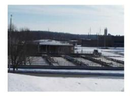
**Polishing Filters** The polishing filters are the next step in the treatment process. They are designed to remove any remaining suspended solids from the wastewater. The filtration media is sand for one portion of the plant, and mixed media of various sizes of sand and coal for the other portion of the plant. As suspended solids are removed from the wastewater, the filter media becomes dirty and the water cannot flow through the filter as fast.
