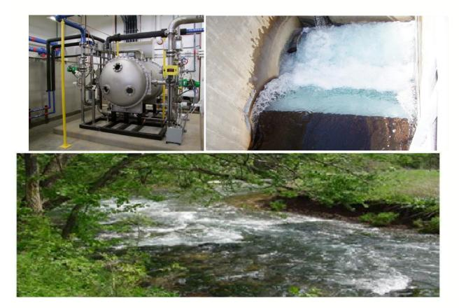
Both liquid and gaseous oxygen with greater than 95% purity can be produced. The liquid oxygen is stored in two 25,000-gallon tanks for use when gaseous oxygen cannot be produced. The Cryogenic Oxygen (CRYO) generation plant can produce 50 tons of oxygen per day.
