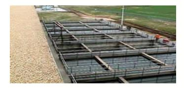
**Ozone Contactor** The flows from the 2 treatment systems come together again for disinfection, the last step in the treatment process. Ozone, which is produced on site, is used as the disinfection agent. The production of ozone consists of 2 stages.
