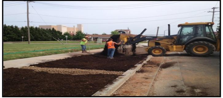
Communicate this to construction staff and/or fence these areas off. Locate staging areas and stockpiled material away from these areas. Compacted soils can be remediated by aeration and compost amendments if necessary. If preservation of trees and/or other vegetation will be utilized as a post-construction BMP, make sure these areas receive adequate protection from construction activities as well.
