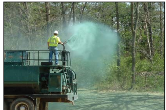
A hydroseeding operation in action.
