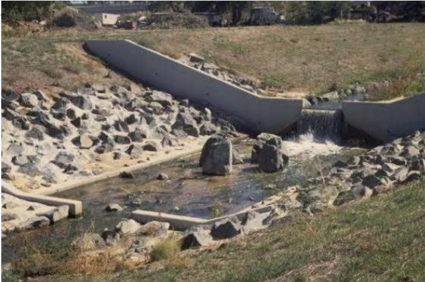
Concrete vertical drop
