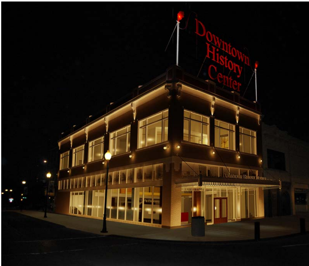
Image of completed renovation project
